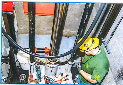
Pictured above, an Otis Elevator technician works on the hydraulic cylinder in the elevator shaft at 408 Adams Apartments.
